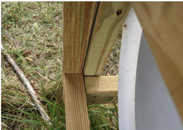
Figure 22. Top view of bottom two (2) 28-inch support planks. Attached to H-shaped legs, sits lower than the 55-gallon barrel half. (Photo Credit: Catherine Terrell)
