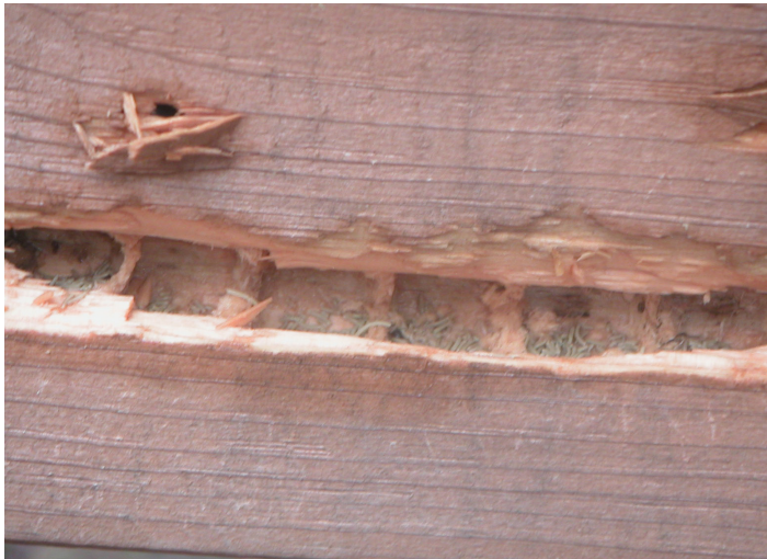
Exposed nest clearly showing the size and the cells created within the tunnel
