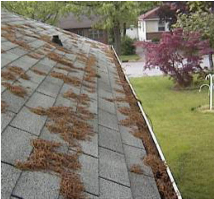
Improperly maintained gutters are habitats for nuisance and vector mosquitoes ( Photo Credit: Purdue University )
