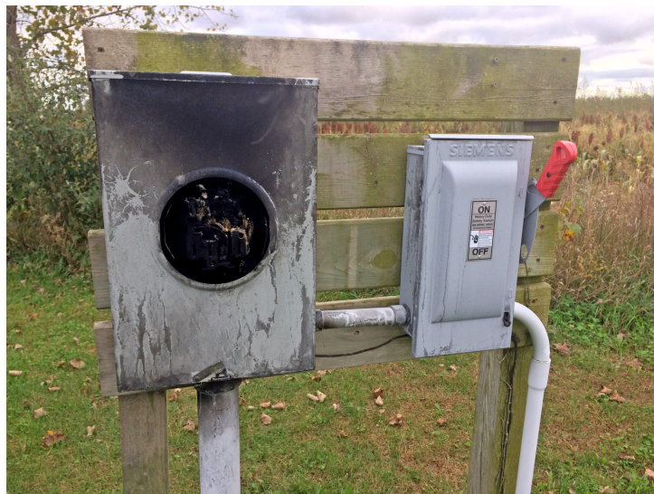
Lightning damage can result in the need for a total replacement of the metering unit and disconnect boxes. The sooner you find the problem, the more time you will have to replace it before irrigation is needed. Photo by Lyndon Kelley, MSU Extension.
