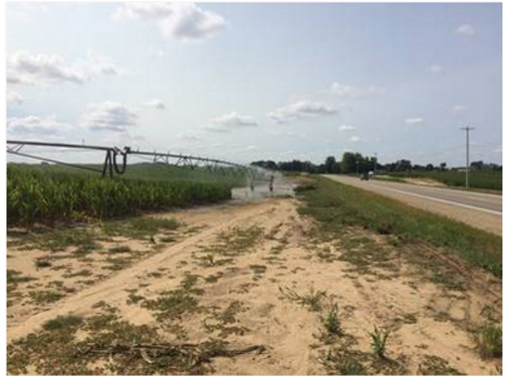
Sprinkler control systems for pivot corner arm are notorious for freeze damage. Proof the system before the season starts so they only water when needed. Photo by Lyndon Kelley, MSU Extension.
