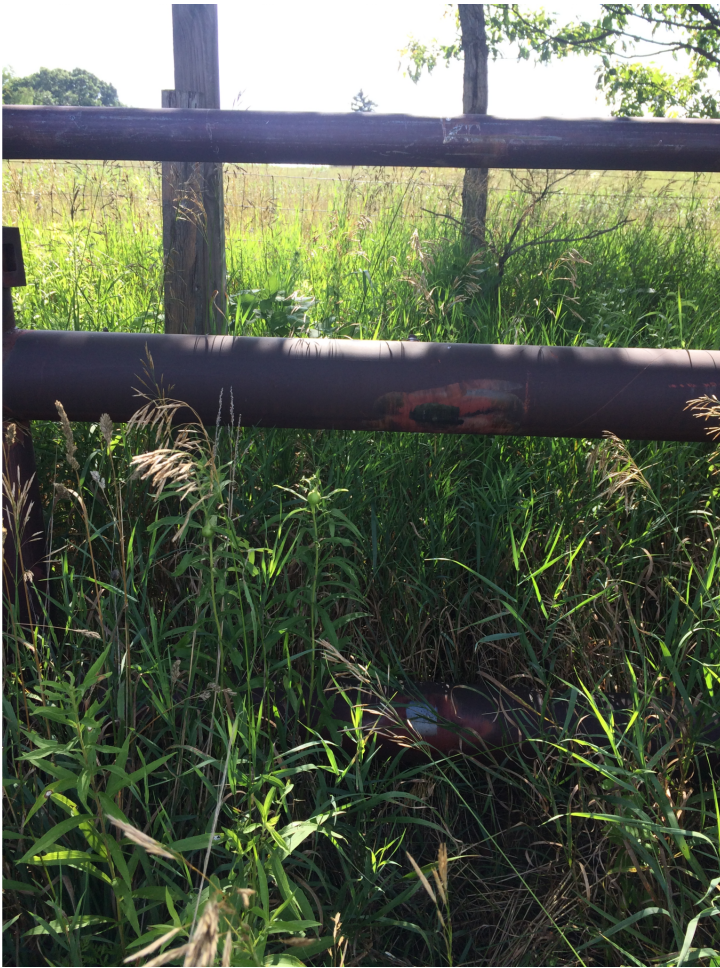
Tire wear marks on the stop barricade indicate the electronic stop has failed recently. Photo by Lyndon Kelley, MSU Extension.
