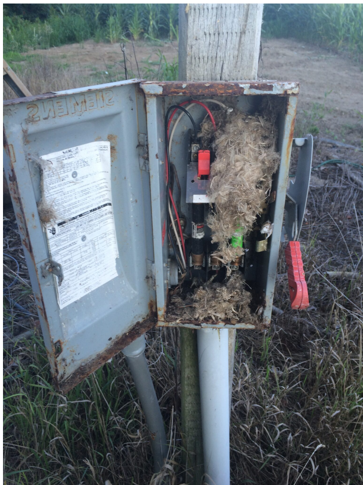
Vermin nests can cause explosions, electrical shorts and corrosion of wires. To avoid a dangerous situation, inspect and clean all electrical control boxes from the power supply to the pivot panel before energizing. Photo by Lyndon Kelley, MSU Extension.
