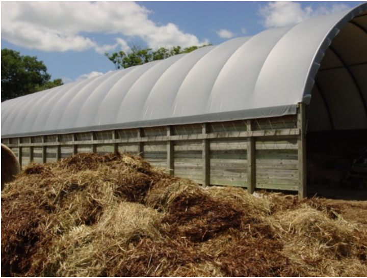
Hay in the foreground was removed from the hoop building because it was smoldering. (Photo Credit: Keith Johnson)
